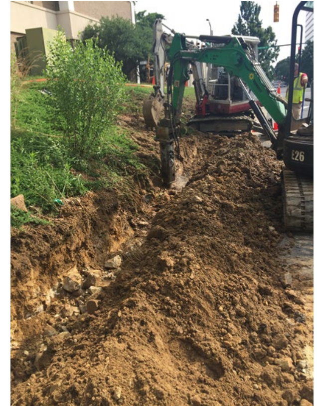
Boring through rock. (schedule and cost increases)
